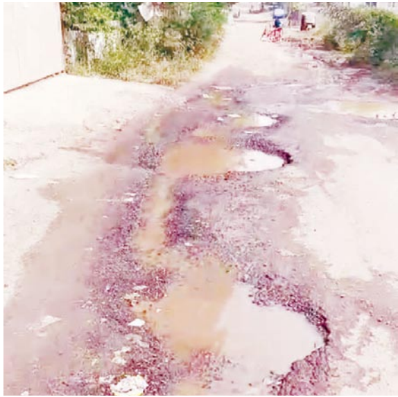
The leak continues round the clock, wasting enormous amounts of water due to the Municipal Corporation's inaction.
